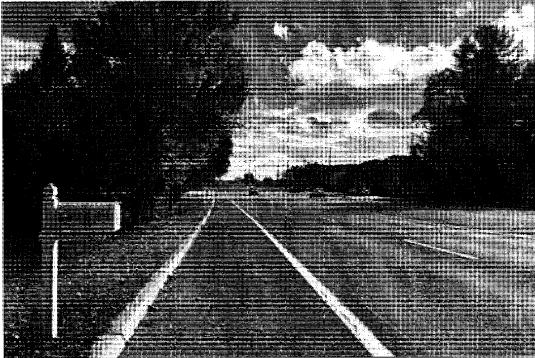
L.O.C.: NYS Route 146 D.O.S.: E Subject: Neighborhood – NYS Route 146 Photo By: E. Stropp Photo Date: 10-19-22
