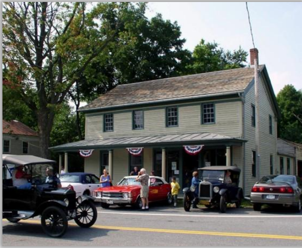
The Historic Grooms Tavern, at the Sugar Hill Road and Grooms Road intersection
