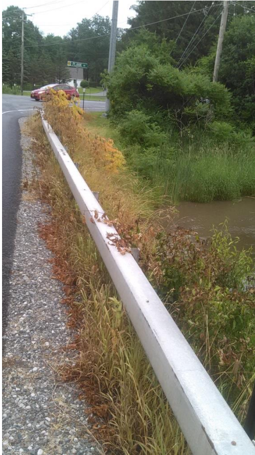
Plank Road at Dwaaskill Bridge
