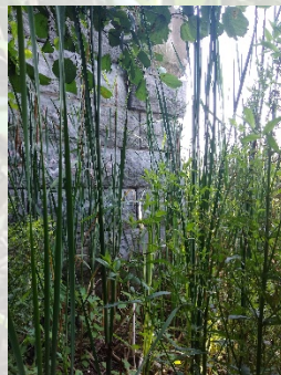
View from below Clutes Dry Dock
