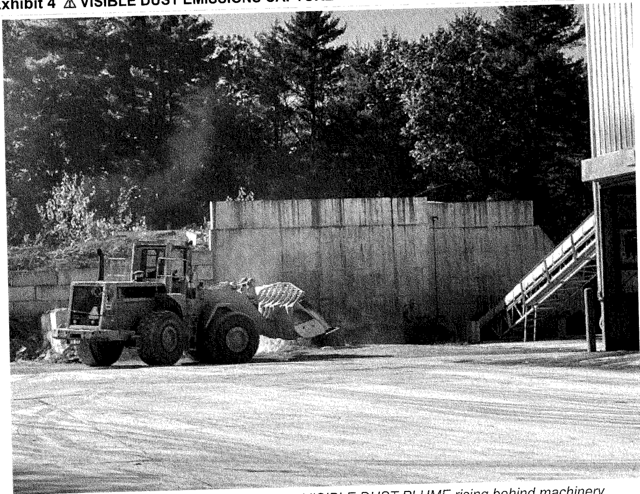
Front-end loader handling aggregate — VISIBLE DUST PLUME rising behind machinery.
