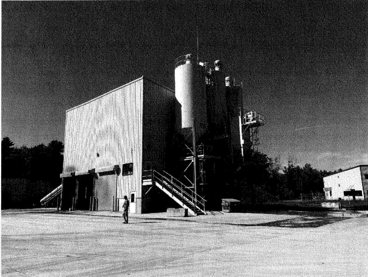
Main batch plant building and cement silos. Person at base provides scale.
