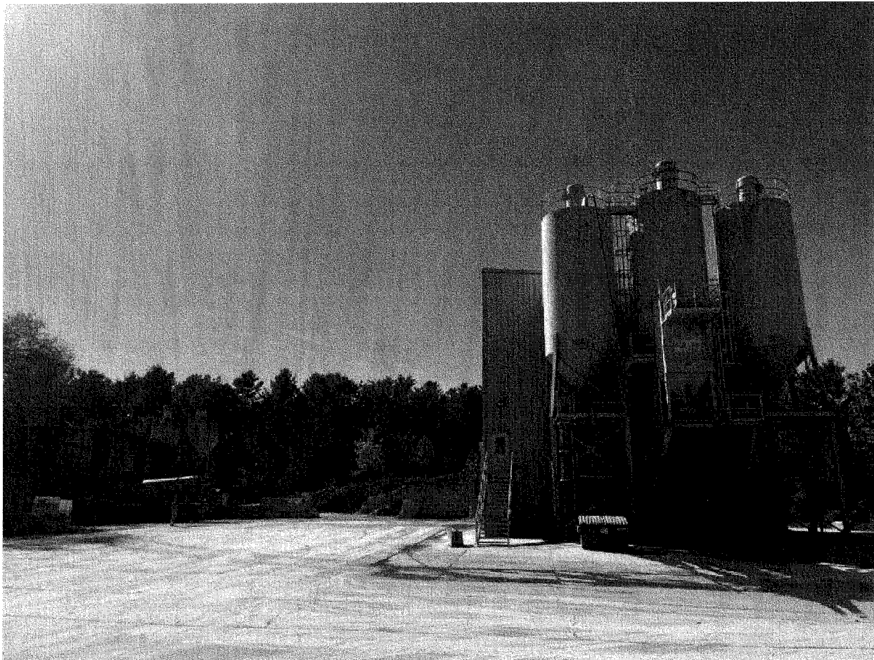
Wide site view showing silos, operational yard, and mixer truck preparing to depart.
