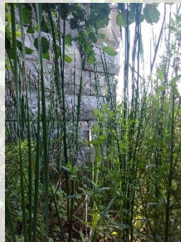
View from below Clutes Dry Dock
