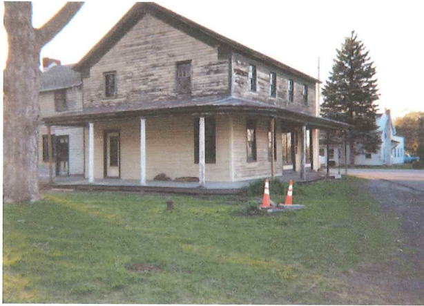
Grooms Tavern at Sugar Hill Road and Grooms Rd. was recently acquired by the town for restoration.
