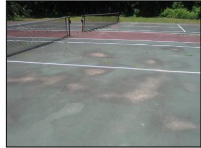
Tennis courts at Clifton Gardens Park
