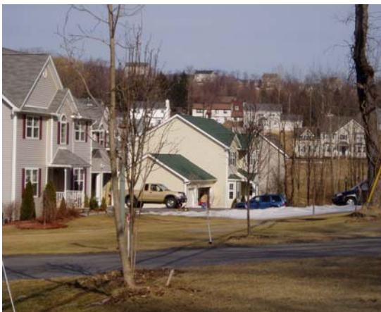
Unacceptable design: note how the homes in the background stick out over the ridgeline.
