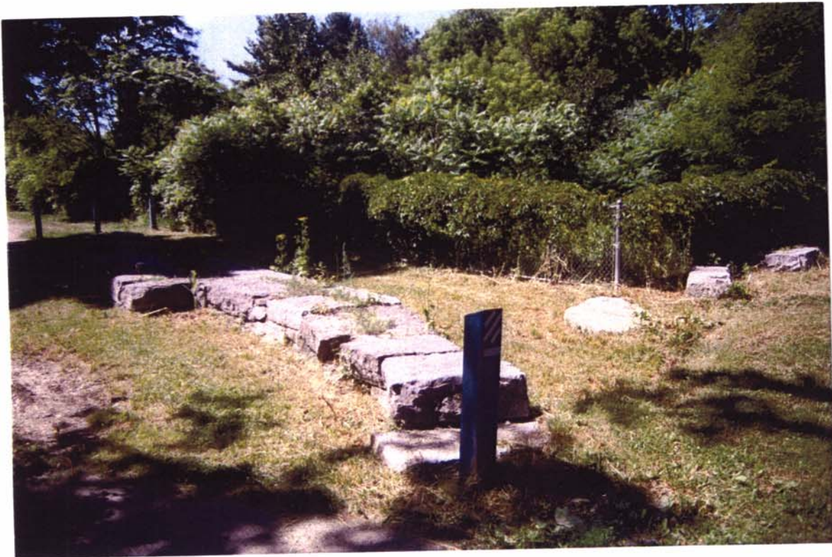
39. Northwest view of canal elements on the north side of Vischer Ferry crossing.
