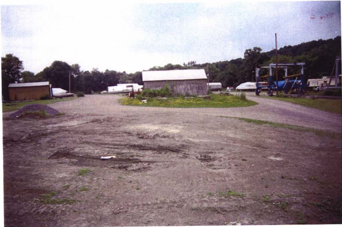
27. West view of a large filled area at the marina.
