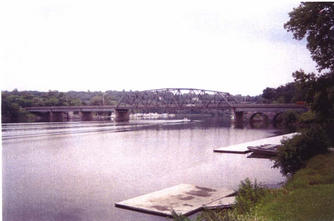
28. Northeast view of the existing bridge, aqueduct, and marina on the river.
