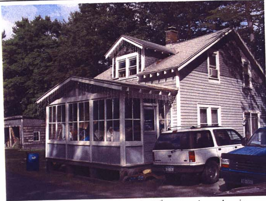
49. 113 East Side Drive. This early 20 th -century bungalow is typical of many of the small houses in Ballston Lake.
