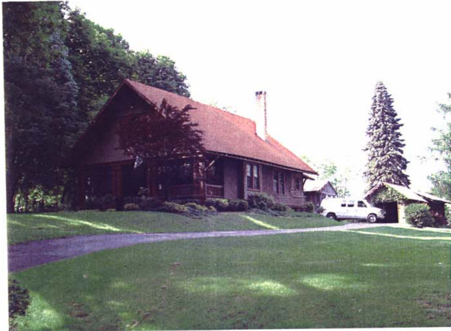
51. 10 Old Schauber Road looking southeast. An example of an early 20 th -century Arts & Crafts style bungalow.
