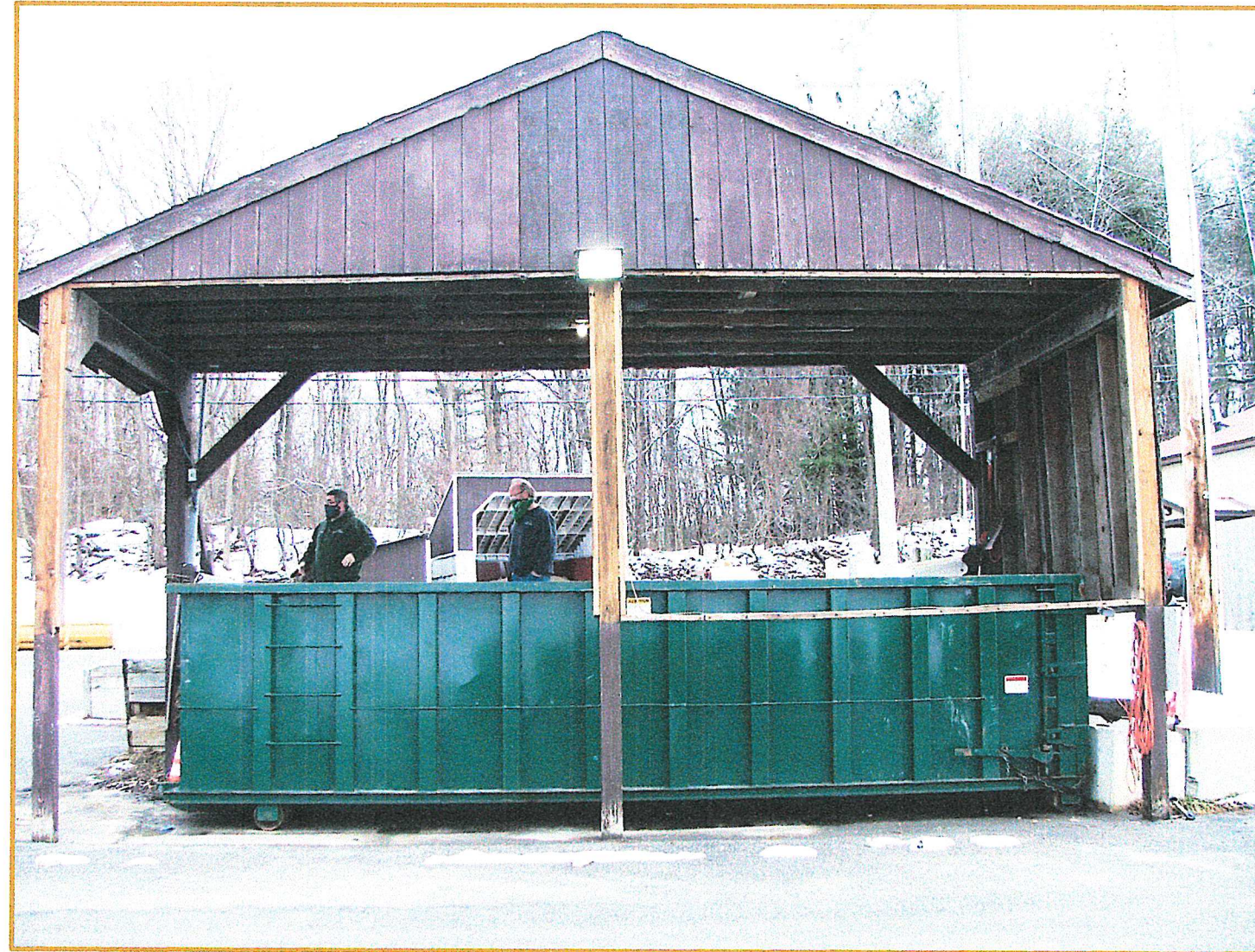
RIGHT SIDE OF EXISTING STATION #4
