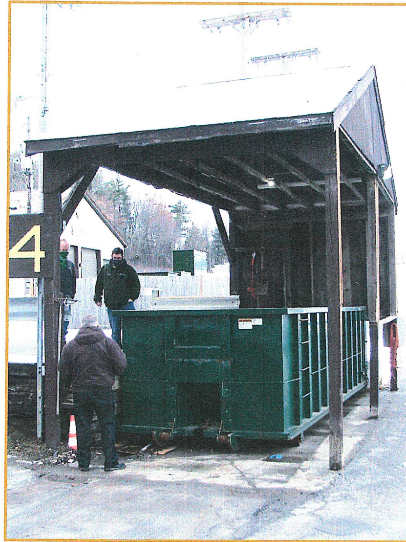
FRONT OF EXISTING RECYCLING STATION #4
